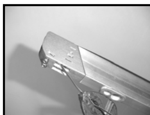
Pull wires taught using a pair of pliers and a vice and screw the wires down on the clamping plate.
